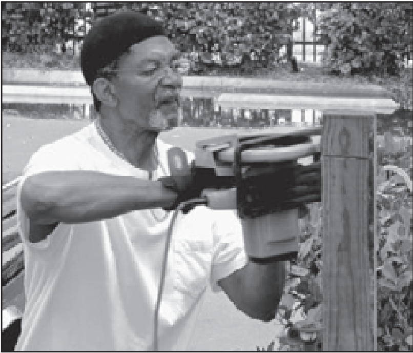
QE Nick Vieira uses a circular saw while building a fence outside the LifeNet4Families building.
